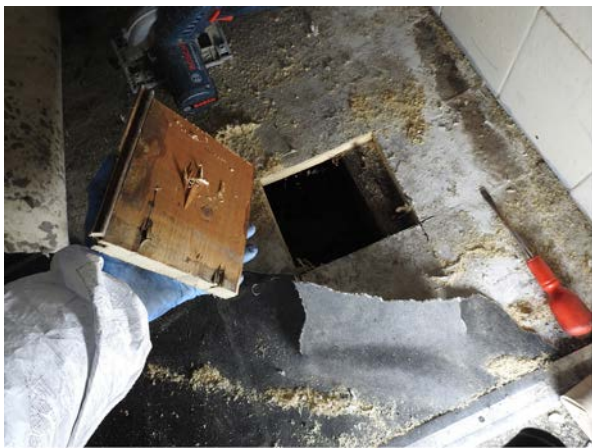
Section of floorboard removed to access ceiling void below
